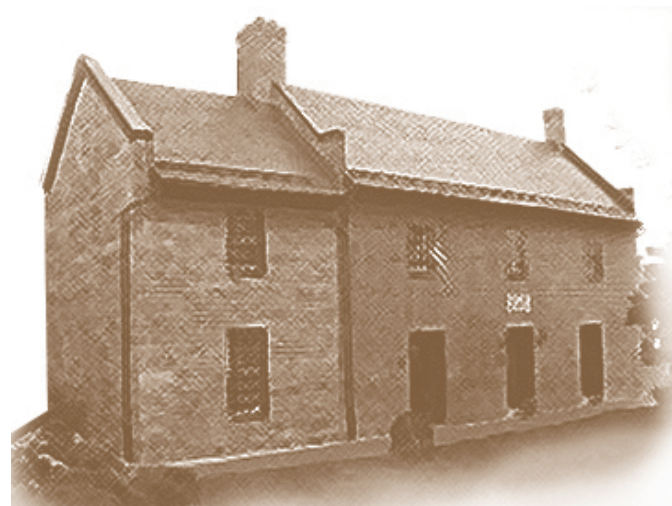
The former Fauquier County jail.
